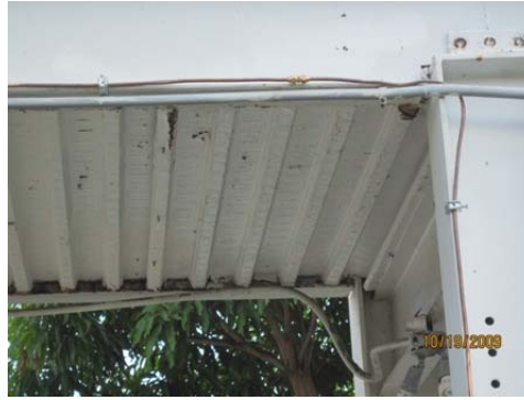
Installed new gas line for new gas tank for pool bar.
