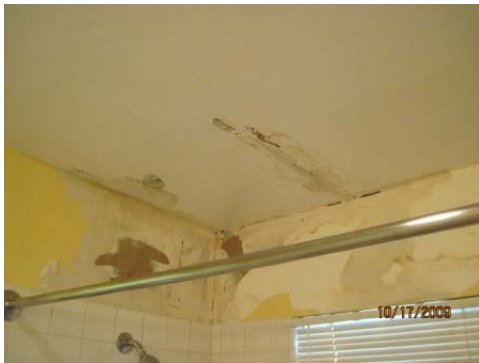
Repaired bathroom ceiling in room 409 from leak coming from room 412
