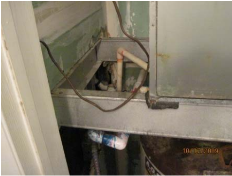
Repaired two more water leaks in room 409, due to brittle piping..
