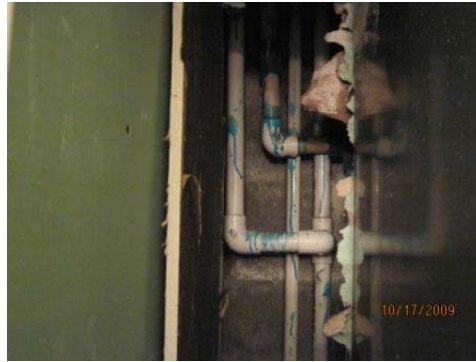
Repaired two more water leaks in room 409, due to brittle piping..
