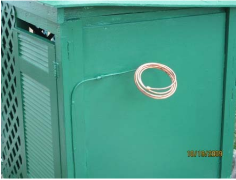
Installed new gas line for new gas tank for pool bar.
