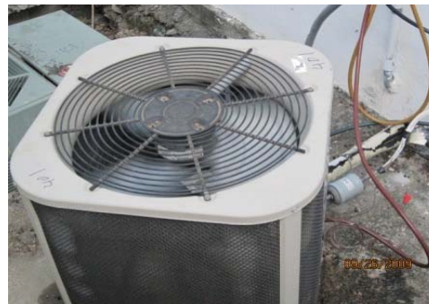
Removed old condensing unit & installing a new condensing unit in room 401.
