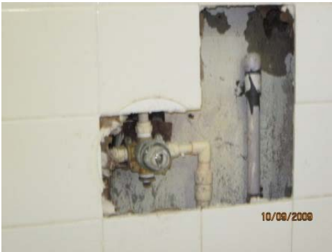
Water leak in Ladies Room poolside shower repaired and re-tiled.
