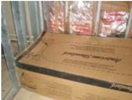
Installation of new Bath Tubs.
