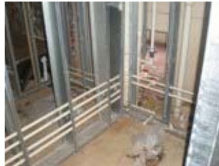
Water piping and metal stud installation.
