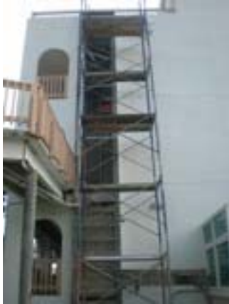
A/C chase demo completed.
