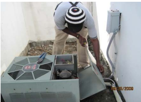
Removed old condensing unit & installing a new condensing unit in room 401.
