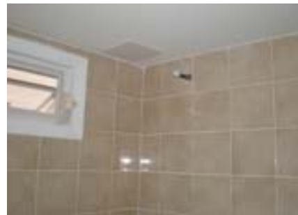
Final touches to tile and plumbing fixtures.
