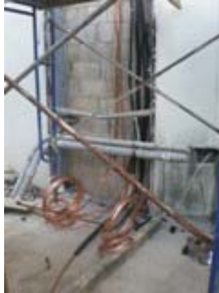
A/C condenser lines being installed.
