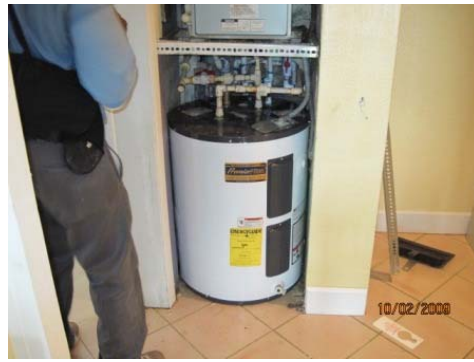
Removed old water heater and installed a new one room 401
