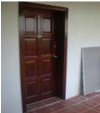
Entrance doors and trim complete.
