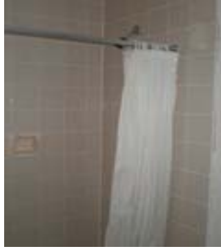
Ceramic Tile completed on 1 st floor
