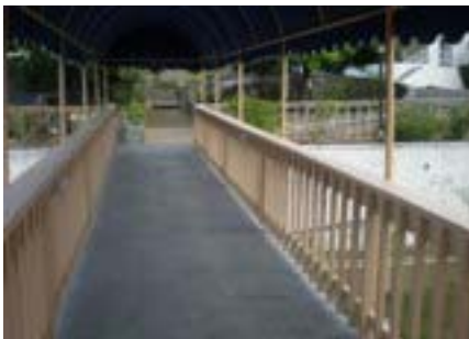
Exterior handrails painted including steps.
