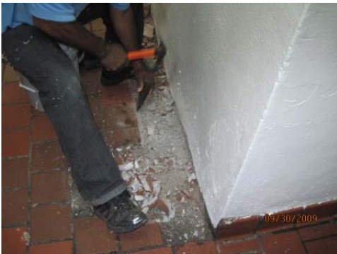
Demolition of rough, broken tile and leveling area. Installing new tile and grout.
