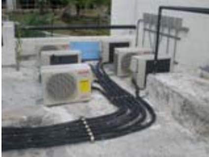
A/C condenser pads complete.
