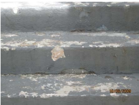
Scraping peeling paint on steps and walkways, and applying non-skid surfacing product.
