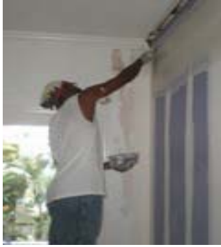
Drywall finishing on 1 st Floor
