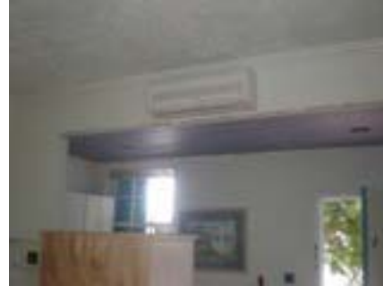
Sheetrock and A/C work on 2 nd floor.
