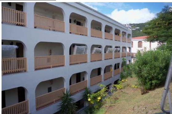
NEW MATTRESSES BEING INSTALLED
