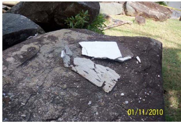
Area of concrete siding which fell from top of the building and landed below
