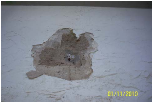
Area of concrete siding which fell from top of the building and landed below
